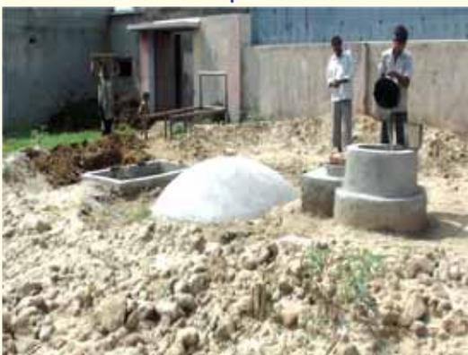
30: Biogas unit in FSR project of PDFSR – Efficient use of cow dung for kitchen gas, lightning and slurry as fertilizer
